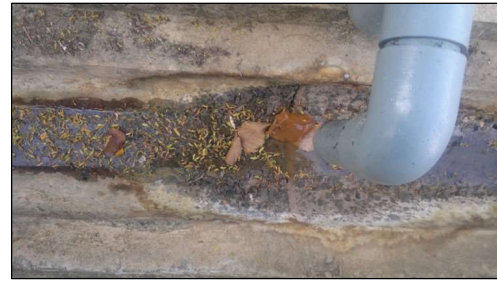
Figure 8. Concrete drain badly corroded by acidic discharge from pre-scrubber and biofilter drain.
