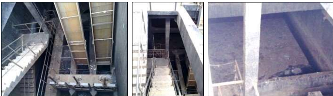
Figure 5. Onsite inspection showed the incoming sewage contain high oil and grease contents.
