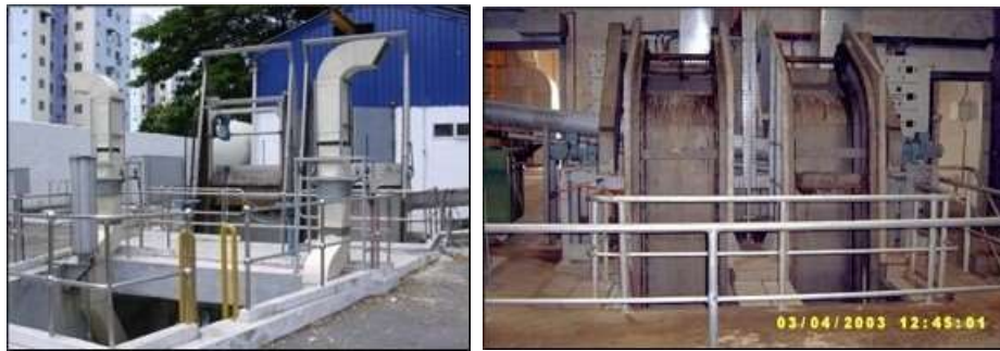
Figure 1. Typical Sewage Pumping Station in Malaysia without Odour Control System
